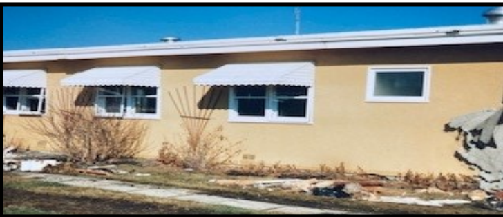
Separating the building from the foundation
