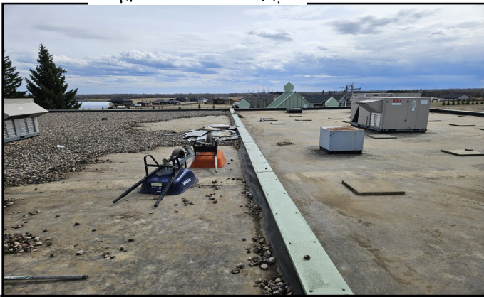
Started on the roof of the church. Completion is happening now.
